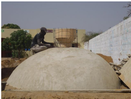
Figuur 27: Houten bekisting ingang vergister
