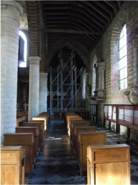
Illus. 2.2: supported vault, beguinage church, Diest.
