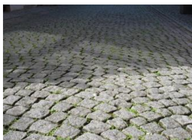
Illus. 2.8: modern paving in Mechelen.
