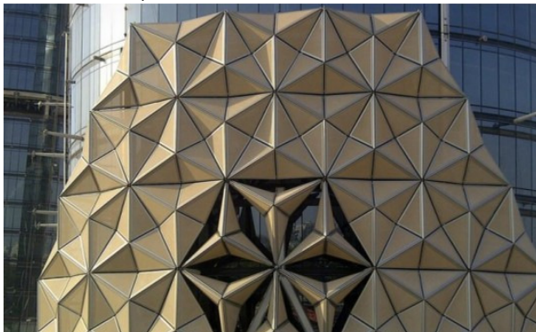
Fig. 17 Adaptable skin of the Crystalline Towers in Abu Dhabi [31]
