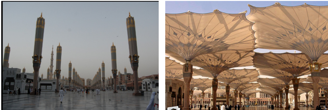
Fig. 14 Foyer of the Masjid Nabawi Mosque in Jerusalem (a) with closed umbrellas and (b) in fully opened configuration in order to provide shading [18]
