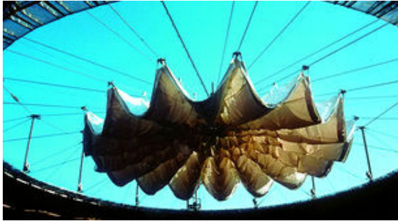
Fig. 15 Opening roof of the bullring in Zaragossa [23]
