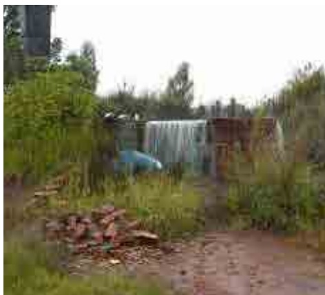
Decant of AMD in the Western Basin
