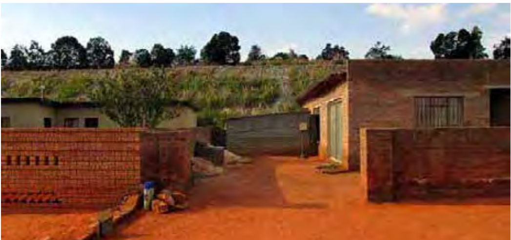
House in Kagiso right next to IL 13-15
