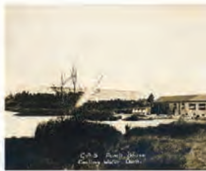
1935 - pump house and cooling water dam (source: Gold One archive)
