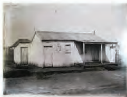
1900 - mine worker's house (source: Krugersdorp Museum archive)
