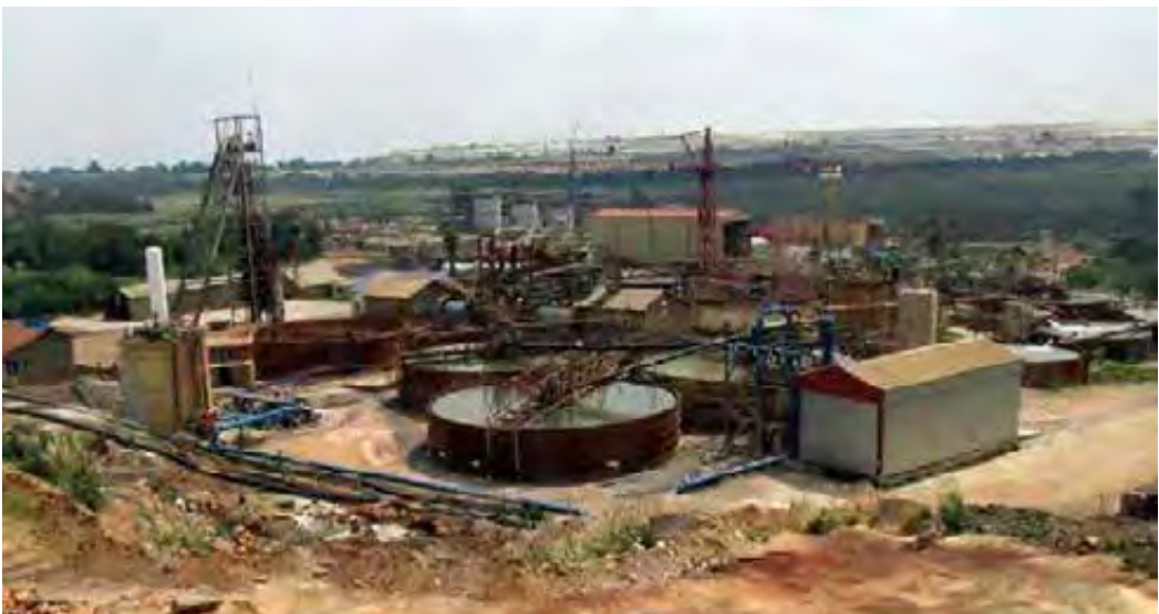
Water treatment plant Mintails (2014)
