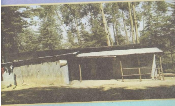
Figure 17: Mosque in Addis Ababa made from steel plates and branches.
