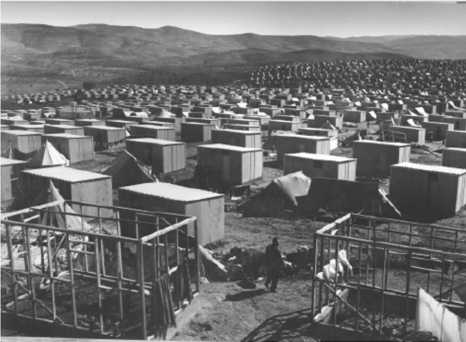
Replacement of tents by asbestos units.
