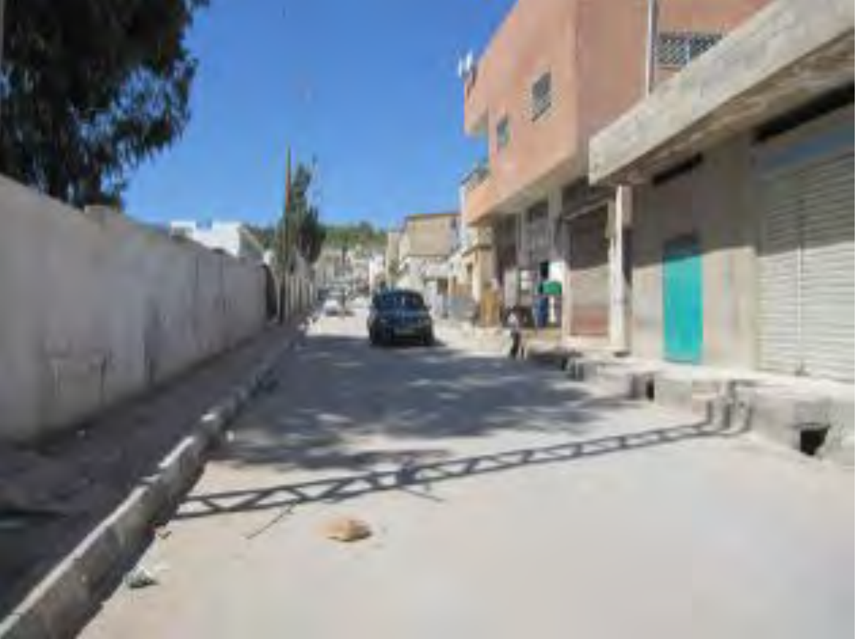
Wall of the UNRWA-compound
