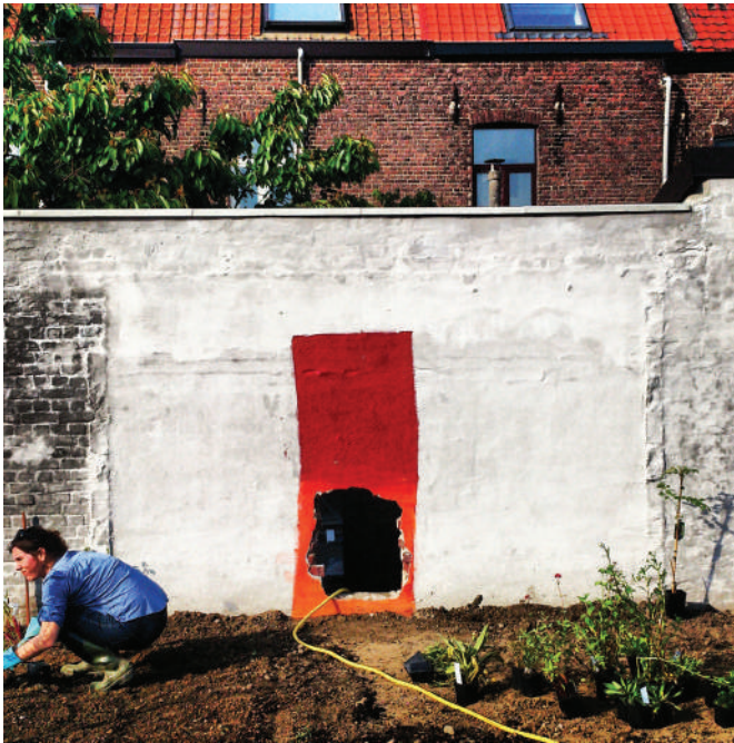
Cautiously breaking through the wall, planting in the garden addition. – May 2014
