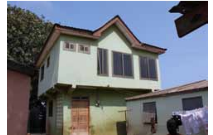
Residential storey building in Tema New Town.
