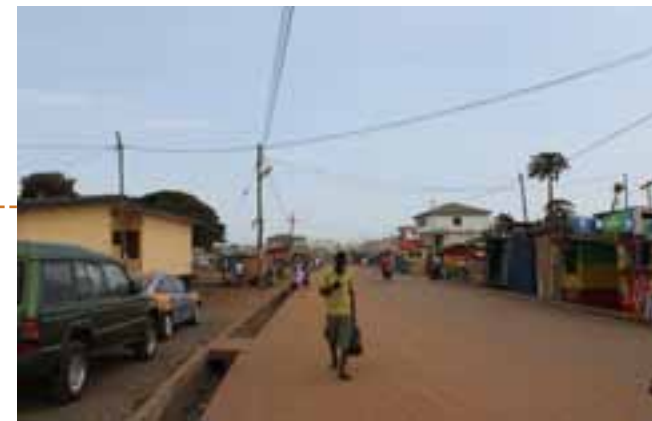
The peripheral roads in section E are largely paved and equipped with a wide open drain which is covered at some places.
