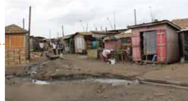
Informal gutter, contaminated with liquid and solid waste.
