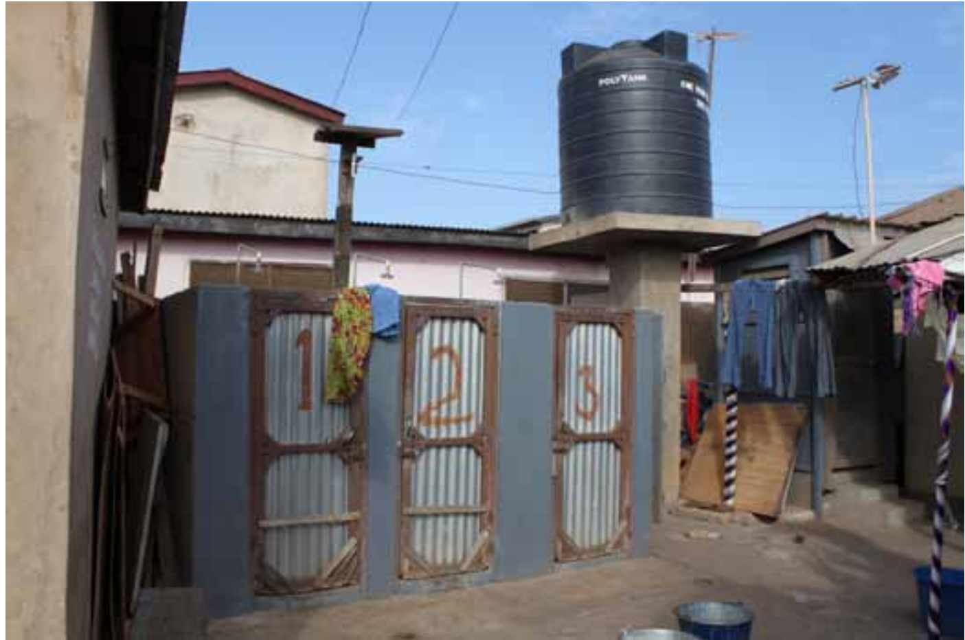
Showers constructed inside the compound of a provider in the low-cost area.
