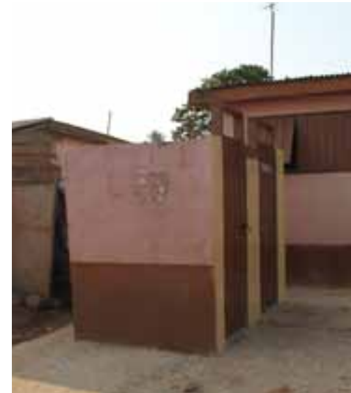
Shared neighbour toilets.
