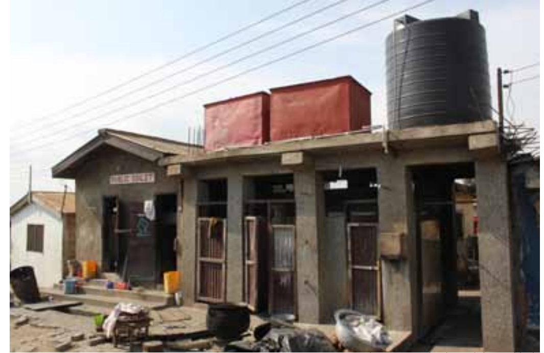
Large-scale commercial toilet and shower block.
