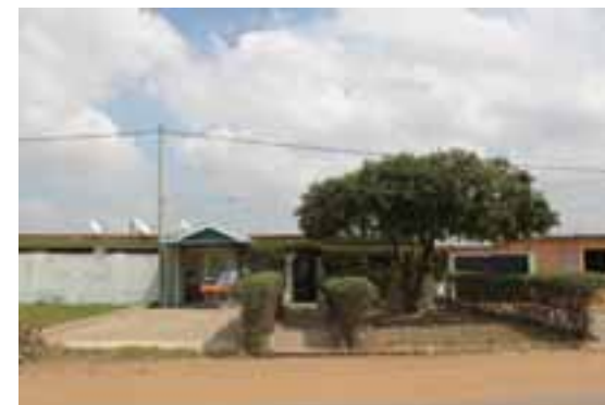
Third phase houses where TDC and TMA intervened when members extended their houses, but as the Society assured the authorities, almost none of them encroached on public lands.
