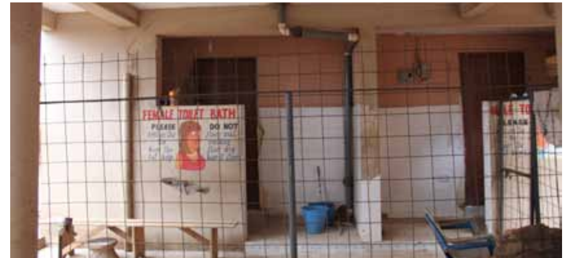
Public toilets and showers in the courtyard.
