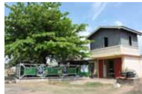
Complete second storey.
