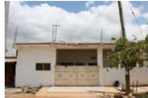
Rooftop covering under construction.
