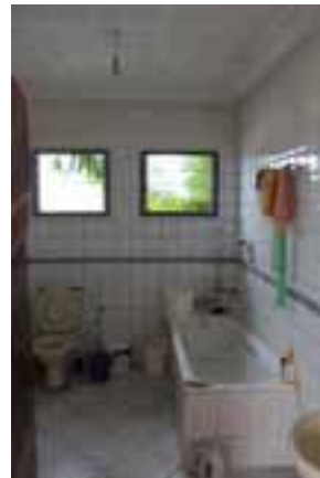
Modern bathroom in a three-storey house in the low-cost area. (C/658A)
