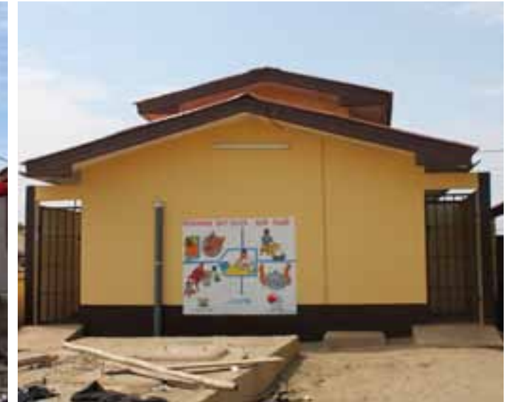
Newly built ASHMA toilet facility.
