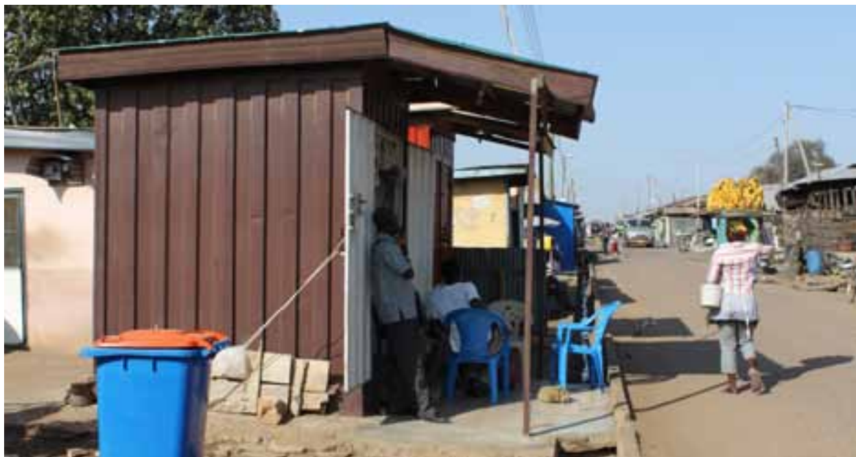
He built two container-shops in front of the house for himself and his son. The space in front of the shops is cemented up to the street border, locally covering the gutter to enhance accessibility.
