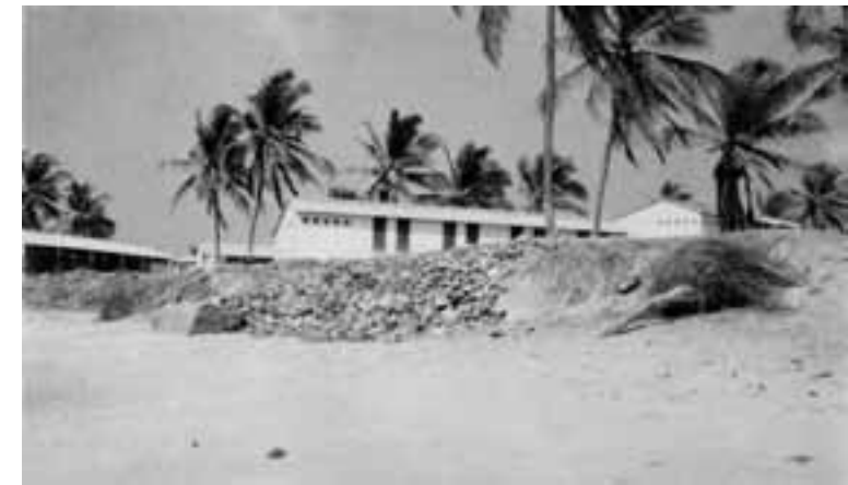
Erosion on the beach. The stones have been dumped by TDC in an attempt to protect the coconut trees.
