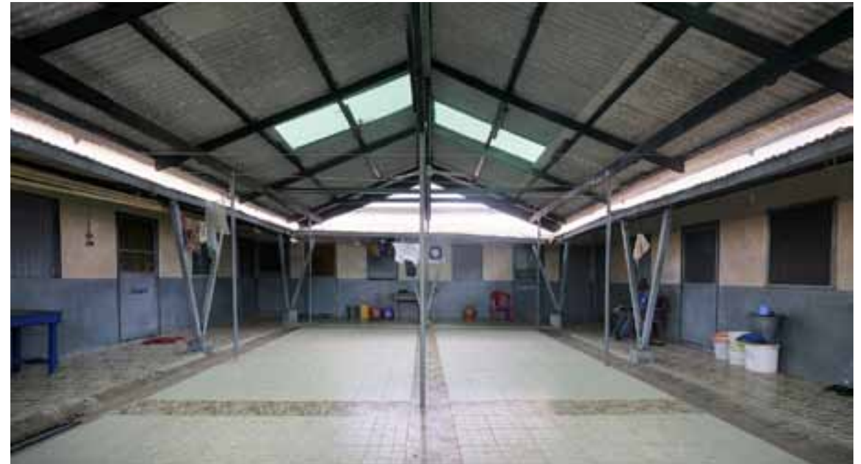
The courtyard was roofed in 2011 and tiled in 2013. Oko Adjetey, one of Obuor We's 'great people' is an architect and designs all the family's construction plans. © Luigi Caterino
