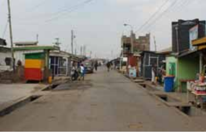
Paved and equipped with gutters.
