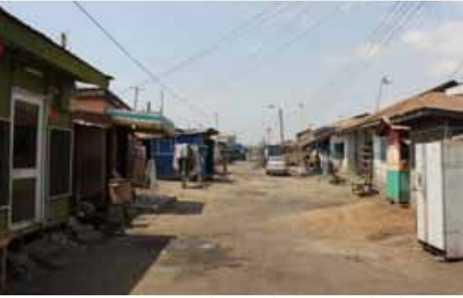
Neither paved, nor equipped with gutters.
