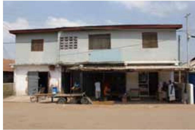
Mixed storey building in the low-cost area of Ashaiman.
