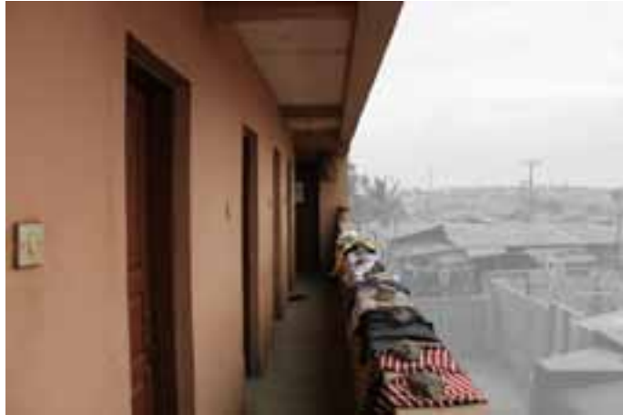
Corridors are used to dry clothes.
