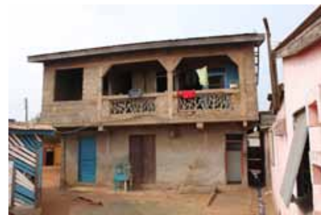
Two-storey extension of a compound in Tema New Town. A veranda or open-air hallway is included where the dwellers can access their rooms and dry their clothes. On the ground floor, one separate bathroom is provided for the residents of the main compound. (D12)
