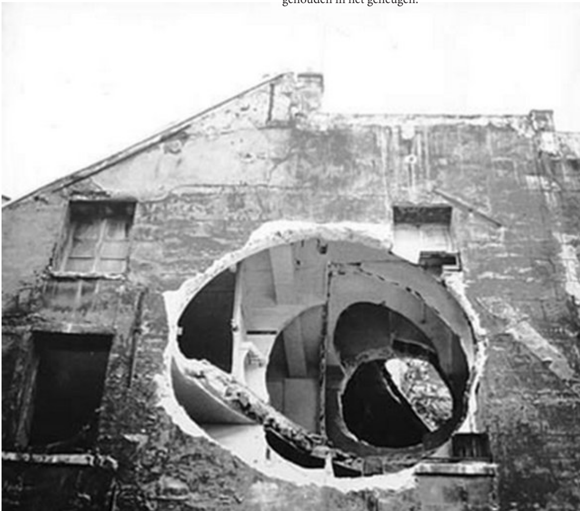
Gordon Matta Clark - Building cuts
