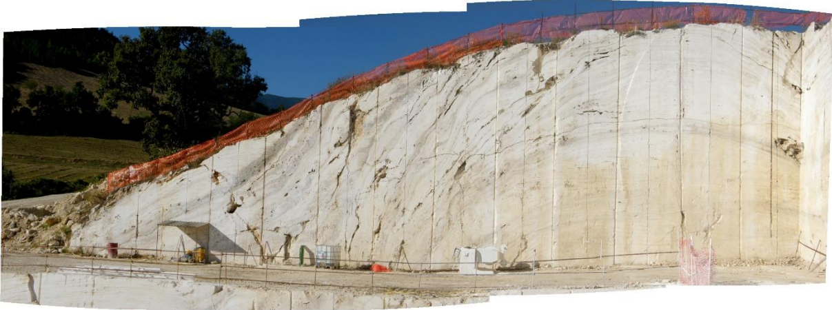
Figure 4-1: Example of a compiled picture of a quarry wall, used in linedrawings and lithofacies variations. Such pictures were available for most quarry walls.
