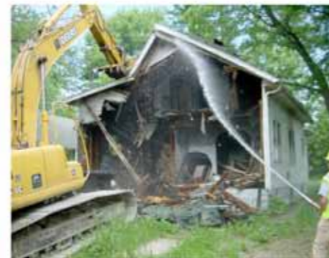
deconstruction project, Kent county, Michigan, US
