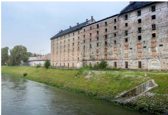
fig 24: canalized river downstream through more harsh environment ('east' Poljane)
