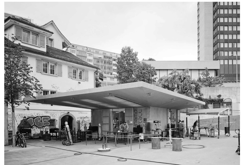
DYNAMO METAL WORKSHOP - PHALT ARCHITECTEN ZÜRICH
